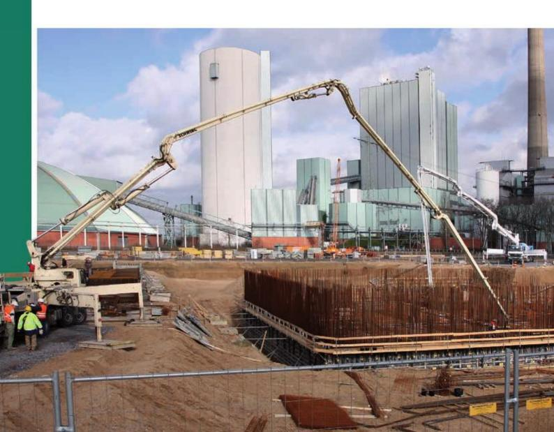
The placing boom puts a range of possibilities at the operator's disposal: its shorter fourth boom segment together with a 200° hinge give this machine optimum slip and threading properties and enhanced mobility.
