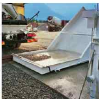
Hydraulic skip for feeding surplus materials from concrete pumps; 1,100 liter capacity.
