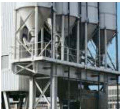
The wide substructure of the cement silos is designed as portal construction. Beside the control container, it can also accommodate social facilities, an admixture tank storage or a heating system.
