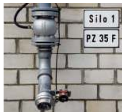
The safety device to prevent overfilling of the cement silo meets the requirements of the UVV. A squeeze valve in conjunction with an optional pressure controller prevents overblowing of the cement silo.
